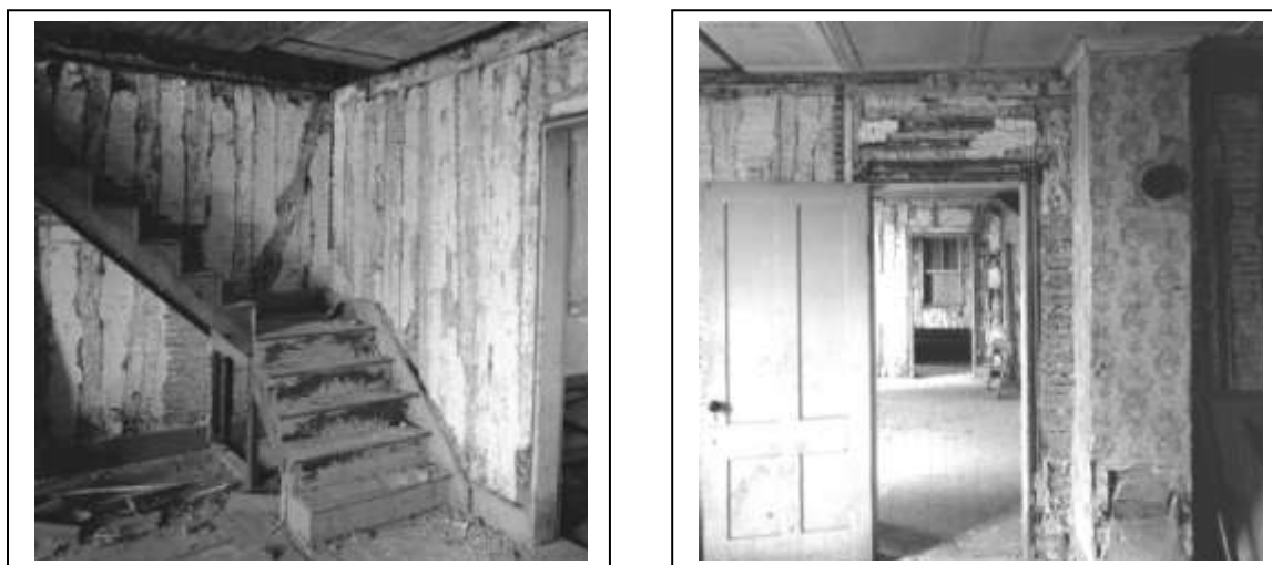
The interior of the house gives clear evidence of its vertical-log construction in the French tradition.
