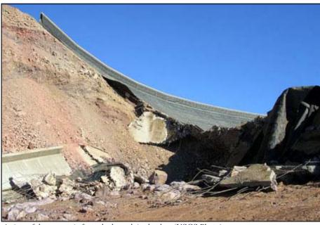
A view of the reservoir from the breach in the dam (USGS Photo).
