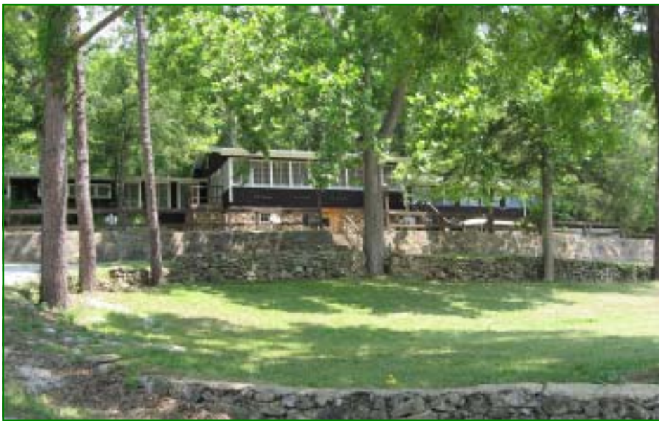
A restored Alton Club Lodge is envisioned as a central focus of a new state park along the Current River.
