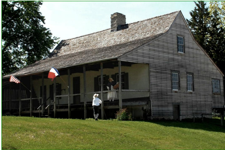
The 1792 Amoureux House will anchor the new National Historic Park.
